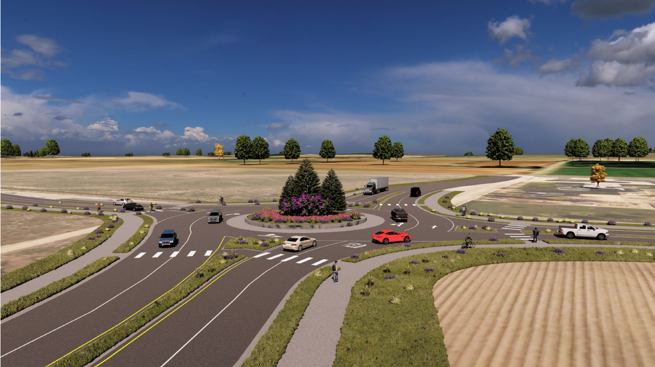
Figure 3.6 – Concept of the proposed two-lane roundabout at the intersection of Meridian Road and King Road
