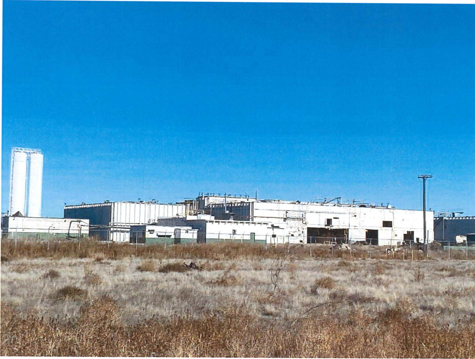
Photo 3. Deteriorating structure within the Kuna East District
